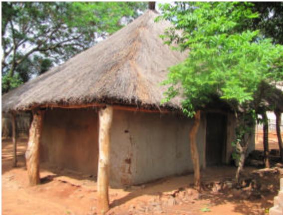
The First SVD House in Mukuni, 1986
